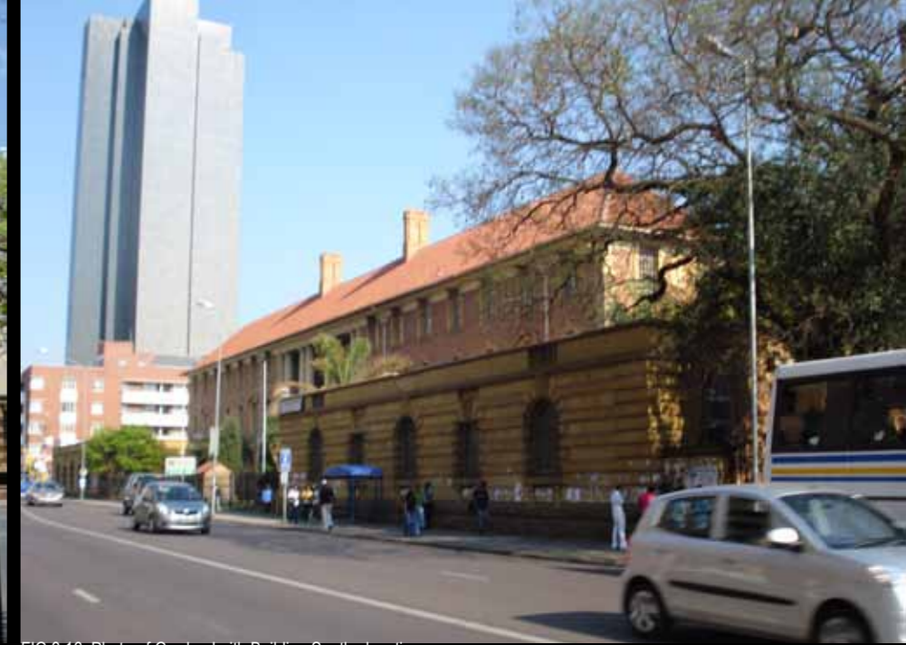
FIG 3.16_Photo of Gordon Leith Building South elevation
