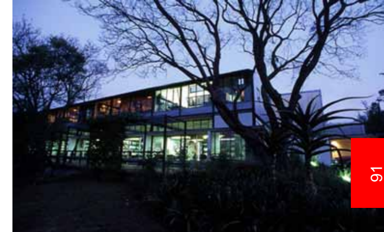
FIG 4.22_Jacaranda trees and steel portal frame solar control on the North facade.
