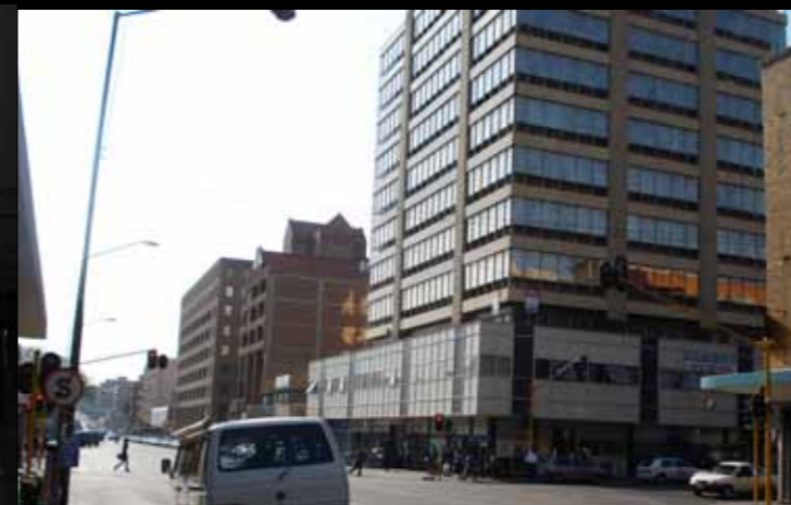
FIG 2.27_SW campus corner facing NE
