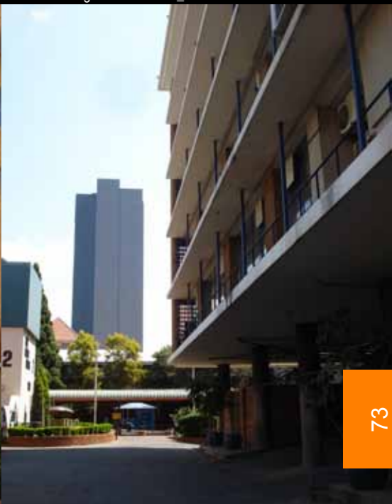
FIG 3.38_Reserve Bank visual axis from Eaton & Louw mezzanine parking
