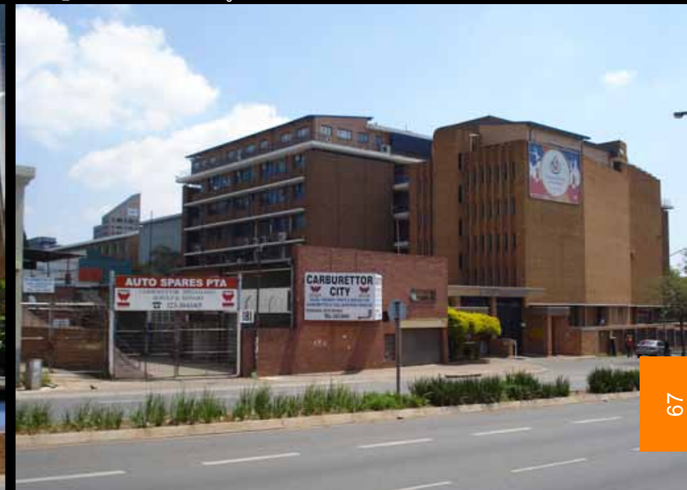
FIG 3.18_Photo of Eaton Louw Building East elevation
