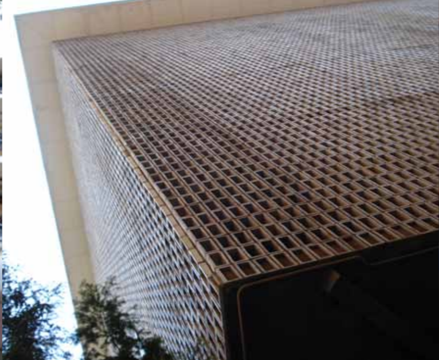
FIG 3.32_Binding Roof Canopy
