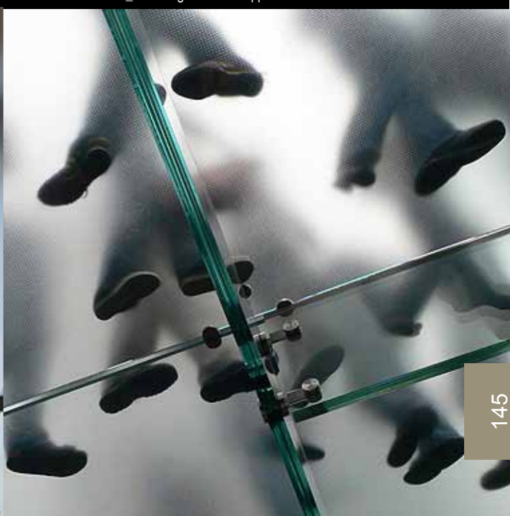
FIG 5.24_Niehaus art gallery roof and sculptural facade FIG 5.27_Frosted glass deck support detail
