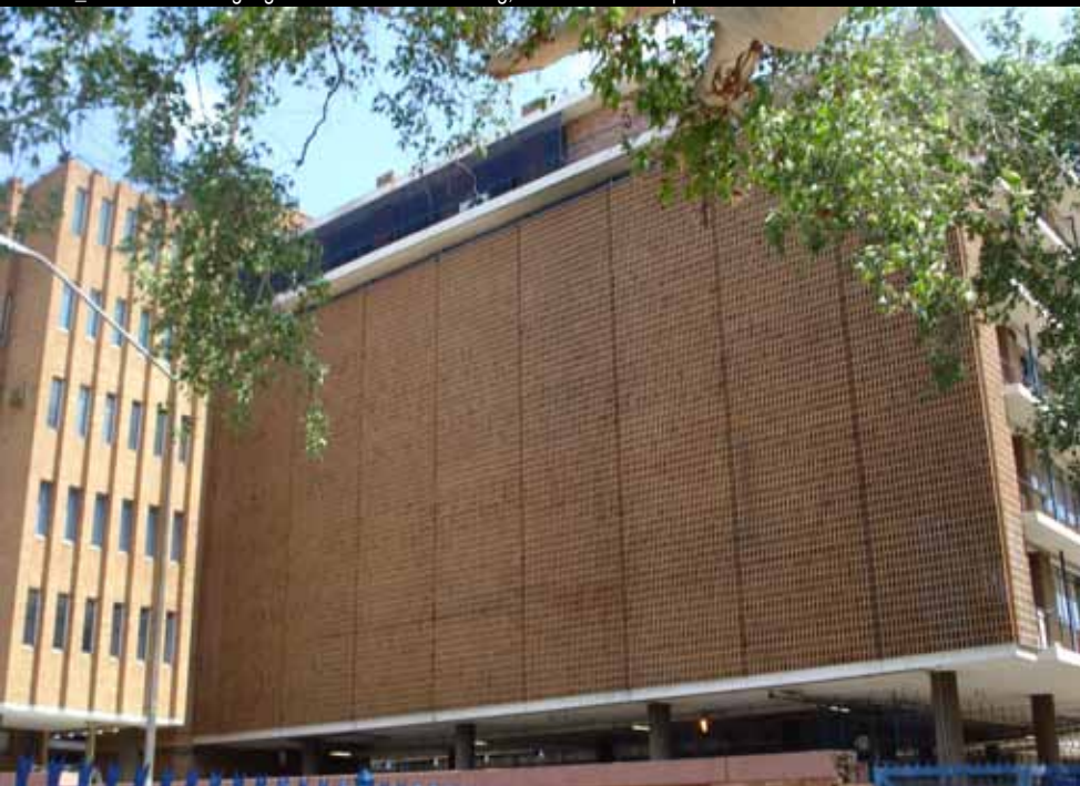
FIG 3.33_NE corner facade of Eaton & Louw Building on Nelson Mandela Drive TUT Science campus
