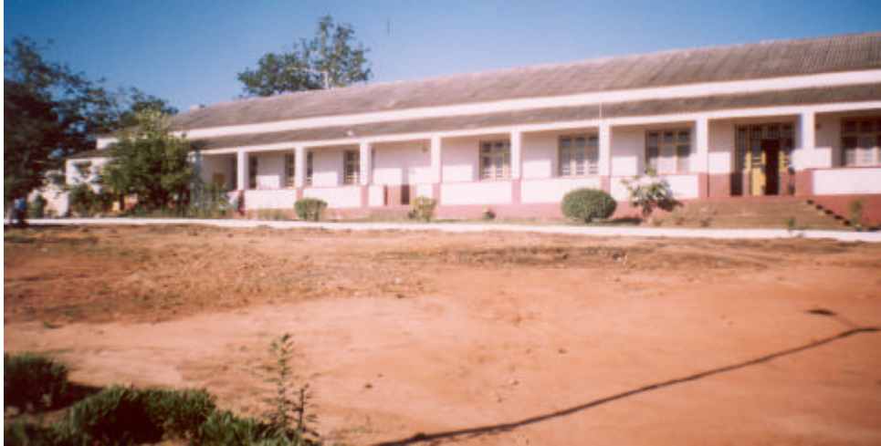
Figure 4.3 Main building – Marrere CFPP
