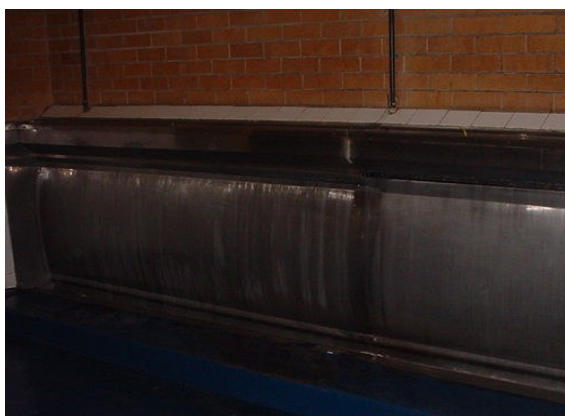
Urinal continuously running
