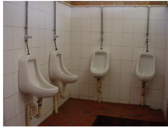
Figure 27:Automatic flushing slab Figure 28:Demand flush bowl urinal
