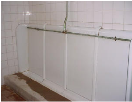
Figure 27:Automatic flushing slab Figure 28:Demand flush bowl urinal
