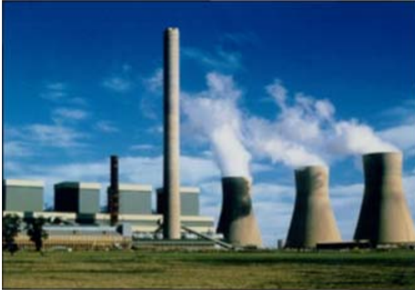
Figure 3.2 A modern pulverised coal-fired thermal power station (Krüger, 1999).
