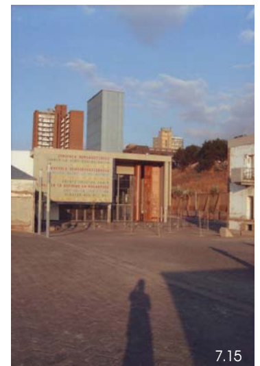
The Constitutional Court Building
