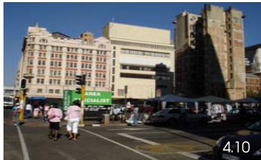
Eastern Edge Of The Site
