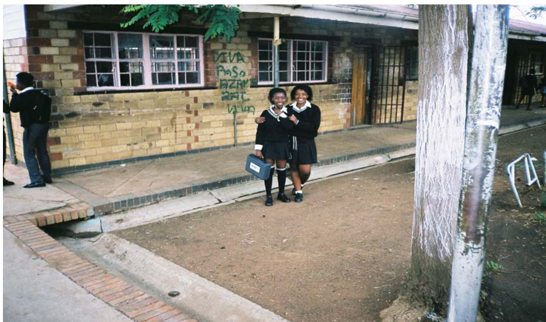
Picture 3: Grade 9 Block, in a state of disrepair
