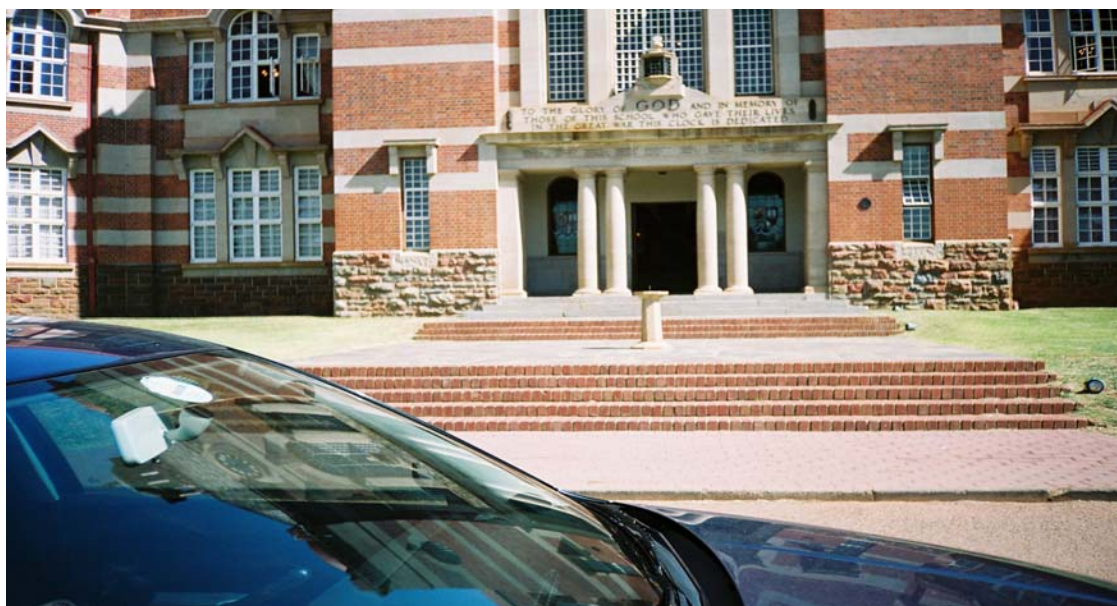
Picture 2: Administrative block. Classrooms behind the building
