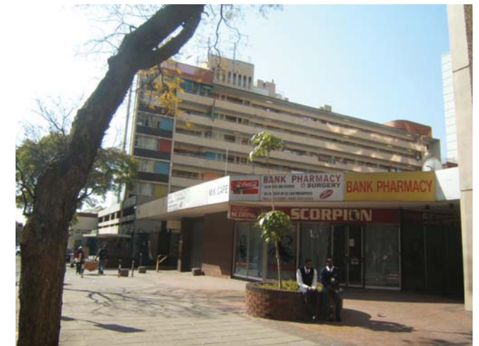
Fig 002.1.11: The “broken” southern façade as it appears in 2010 without screen walls above walkway walls
