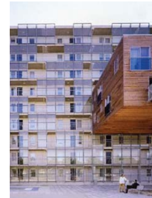
Fig 002.8: Image of northern façade with suspended units employed to optimise sunlight and [re]duce coverage
