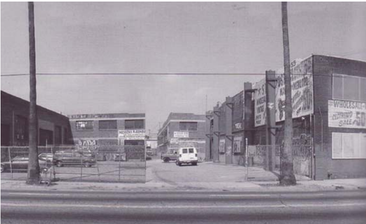
Fig 002.10: The previous street façade
