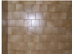
Fig 003.5.21: This tile finish can be found in the lift lobby on the ground floor
