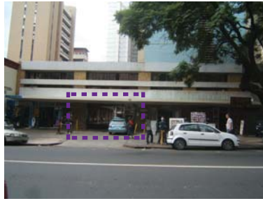
Fig 005.1.1: All office employees and residents need to pass through the opening/ tunnel in front of the blue car
