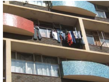
Fig 005.1.7: Residents also resort to hanging washing out the windows on the northern façade. The original clothes lines placed in the bathrooms are inadequate and many have been [re]-moved
