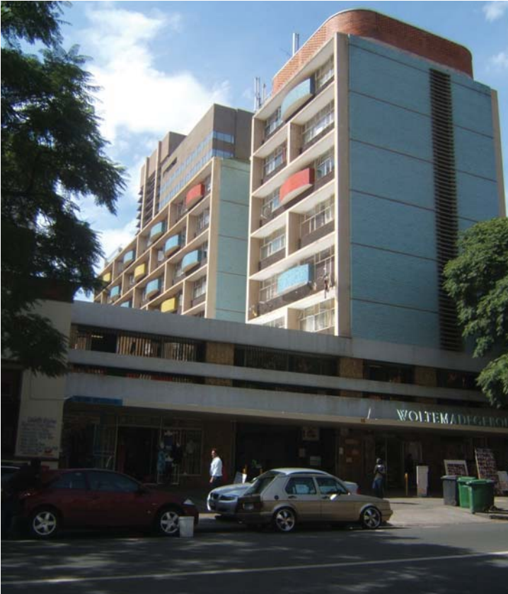
Fig 003.4.4: The western façade is the most prominent side of the building as this is what most people see
