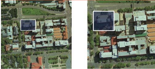
Fig 004.18: Aerial photographs illustrating the site in context
