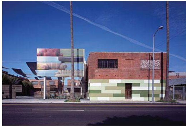
Fig 002.11: The street façade after the [re]novation
