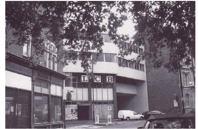
Fig 002.26: The previous street façade of the station sits uncomfortably in its Victorian surroundings
