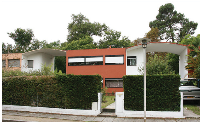
Fig 002.24: The street façade after renovations
