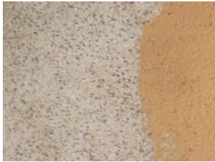
Fig 003.5.4: The block addition on the street edge is finished in gamma zenith which has been painted
