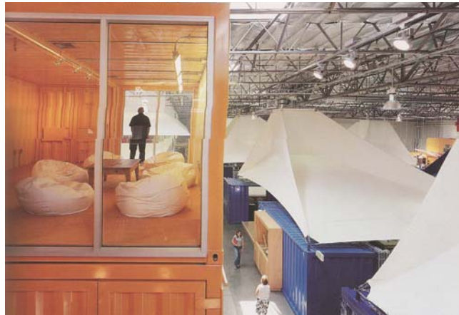
Fig 002.34: Containers provide space for offices and meeting rooms. Tensile structures are anchored to some containers to define spaces
