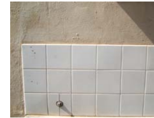
Fig 003.5.25: The walls of the laundry area connected to the building are finished with gamma zenith. White tiles can be found above the wash troughs
