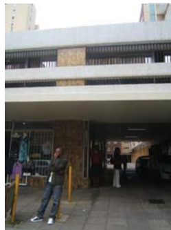
Fig 005.1.4: The middle of the “tunnel” is dark, especially with the lights turned off
