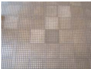
Fig 003.5.19: External walkways on the southern side are finished with the same tiles as the stair landing
