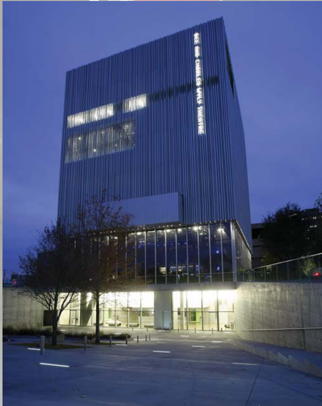
Fig 002.46: A view of the theatre building showing the lobby below with the theatre space above
