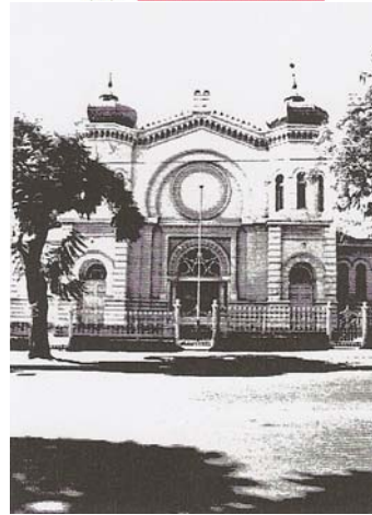
Fig 003.4: Western façade of the Old Synagogue
