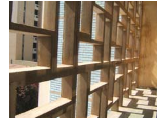
Fig 003.5.12: A concrete screen extends the full height of the building on the northern façade in front of the circulation core
