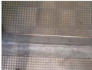
Fig 003.5.18: The transition from inside the lift lobby to the external walkway
