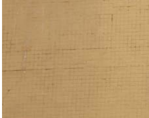
Fig 003.5.5: Upper portions of the block addition have a mosaic tile finish which has subsequently been painted
