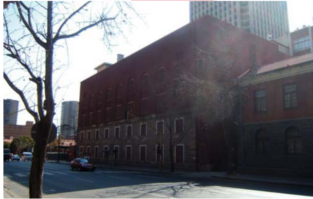
Fig 003.9: The Telephone exchange building on Vermeulen Street
