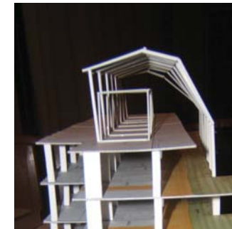
Fig 004.4.24: Steel trusses define space with their change in shape causing a fan-effect along the walkway
