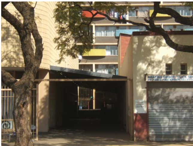
Fig 003.4.10: Here the connection can be seen more clearly. The corrugated roof frames the linear passage towards the Woltemade building, which can be seen in the background
