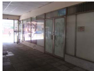
Fig 005.1.9: According to other shop owners, the shop to the rear with blacked-out windows has been vacant for more than a year
