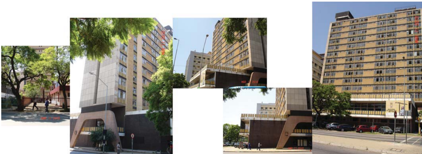
Fig 004.20: Series of photographs illustrating the character of Site 6, starting with the southern most border and moving towards the northern façade
