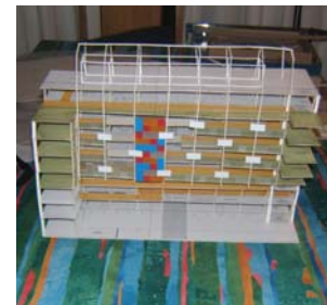
Fig 004.4.22: White, clear, translucent and coloured panels can be seen on the façade
