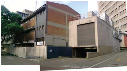
Fig 004.3: Site 1 from the south-west corner
