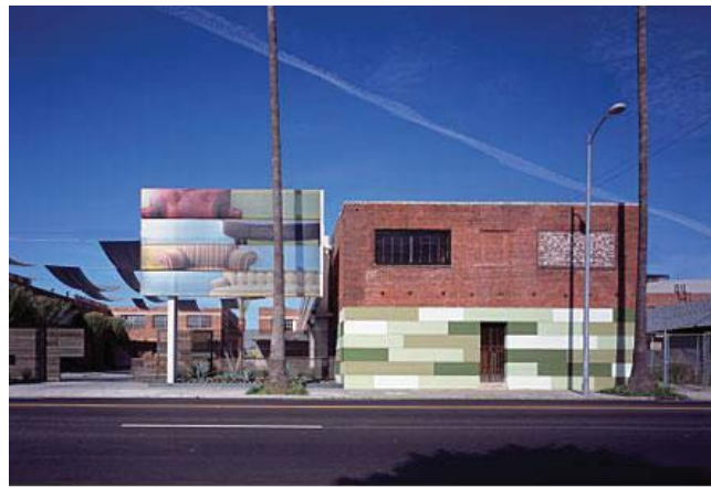
Fig 002.11: The street façade after the [re]novation
