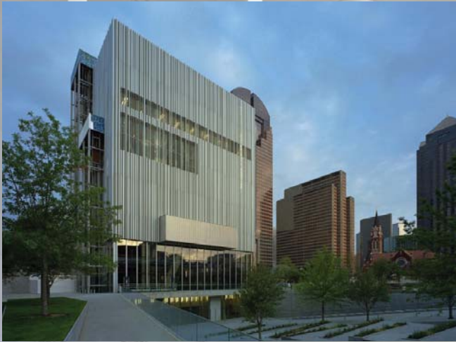
Fig 002.44: This side of the theatre opens up onto a public gathering space
