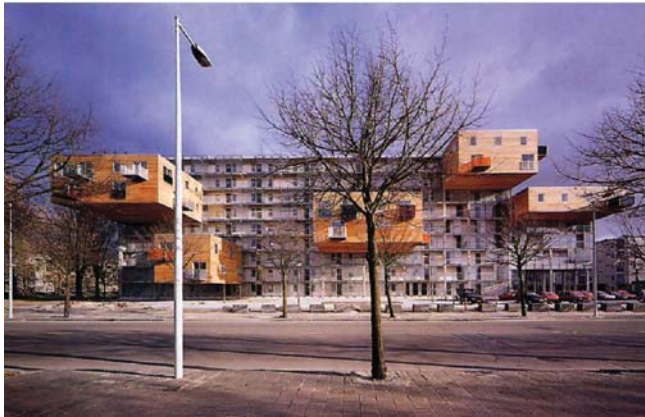
Fig 002.3: The street elevation of the Wozoco's apartment building
