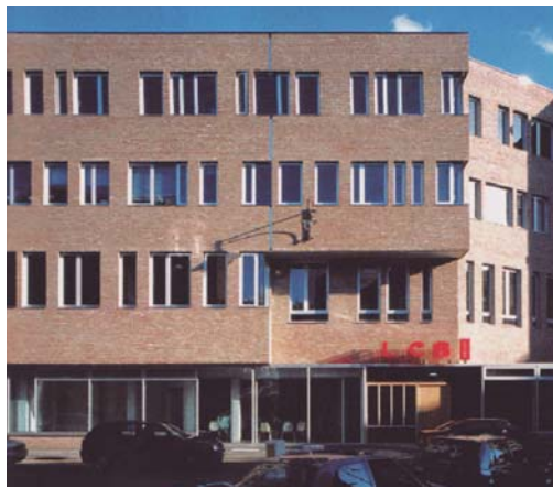
Fig 002.27: The LCB Depot renovated, showing the new facebrick, aluminium windows and café
