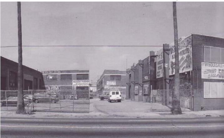
Fig 002.10: The previous street façade
