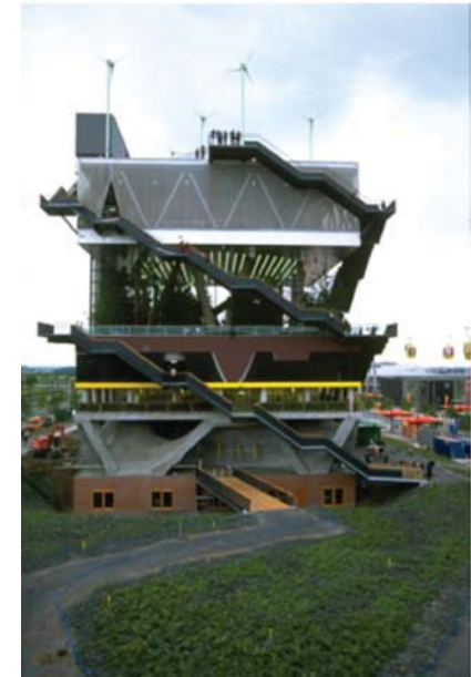
Fig 002.2: The Dutch Pavilion utilises a water [re]clamation system to distribute water throughout the building
