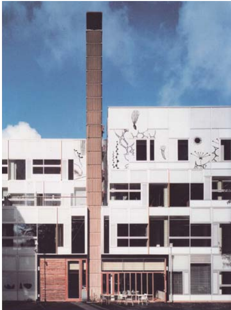
Fig 002.33: The rear of the station building is finished with clear as well as white glass. Some panels display artwork by Linda Schwab
