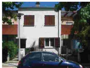
Fig 002.18: The strip window has been [re]placed by rectangular windows with shutters
