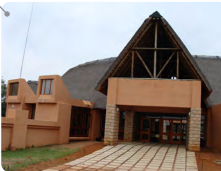
Existing visitor's center Fig. 52
