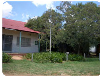
Existing staff housing Fig. 47
