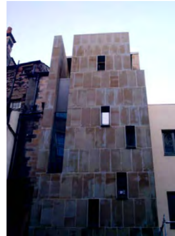
Fig. 67 Scottish Storytelling Centre facade
