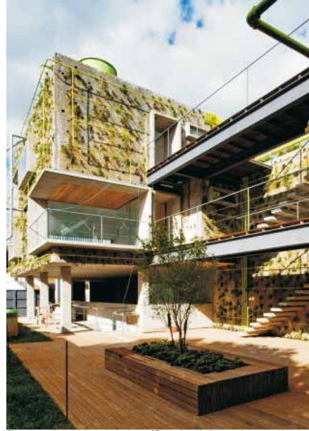
Figure 64. Harmonia office building: the walls are thick and covered externally by a vegetation layer that serves as the skin of the structure: Harmonia 57 by Triptyque, 2008.
