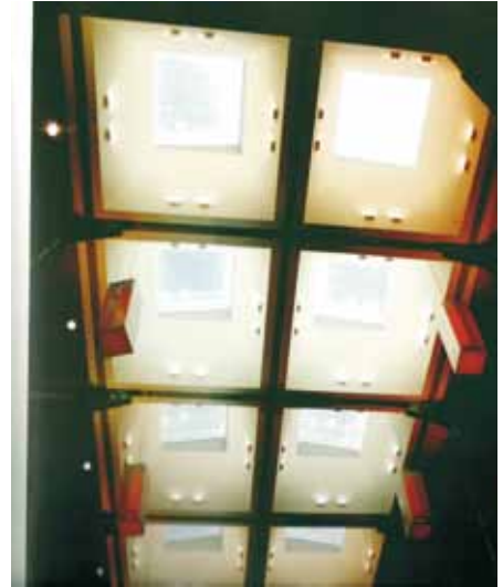
Figure 60. The original concrete hoppers in the demolished North Boiler House are commemorated as skylights in the central atrium of Turbine Hall: Krige & Beswick, 2001: 110.
