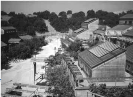
Figure 57. John T Lyle Regenerative Centre: roof profile design to accommodate solar panels:Stine, 2000.
