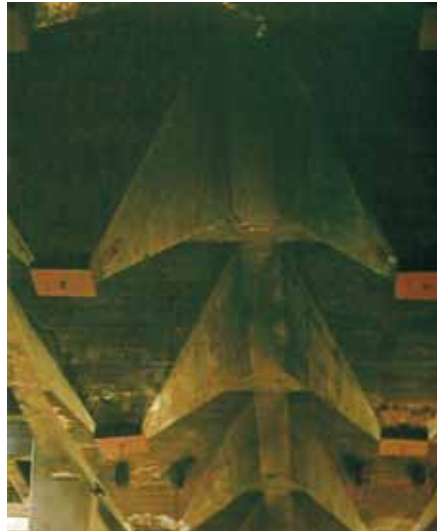
Figure 60. The original concrete hoppers in the demolished North Boiler House are commemorated as skylights in the central atrium of Turbine Hall: Krige & Beswick, 2001: 110.
