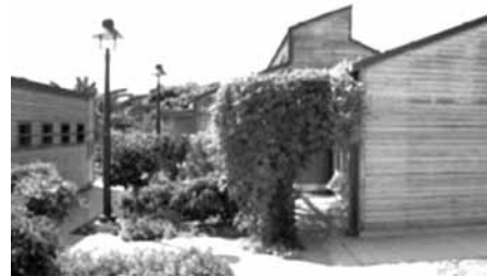
Figure 56. John T Lyle Regenerative Centre: a trellis structure on the southern side of the building support deciduous vines, the shade from the vines blocks direct sun from entering in the summer, helping to keep the interior spaces from heating up: Woo, 2010.
