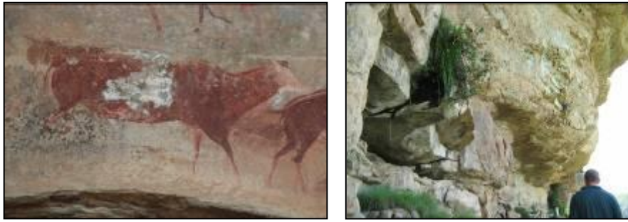
Figure 7.39: Examples of natural deterioration and Game Pass Shelter's rock stability – Left: flaking. Right: Vegetation coming out of the rock surface (Photographs: C.L. Fordred).
