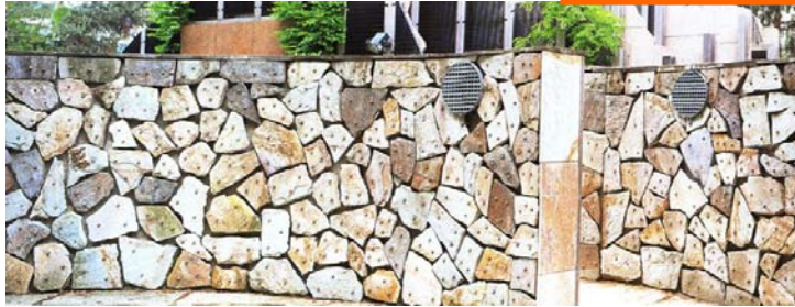
fig.6.44: Wall treatment in underpass
