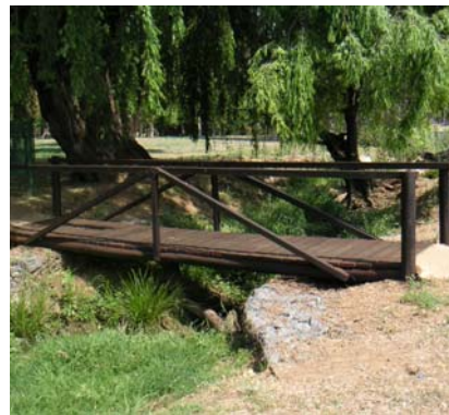
Fig 3-49 Timber pedestrian bridge
