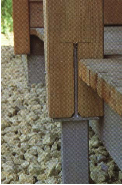
Fig 7-16 Timber and steel - pergola detail
