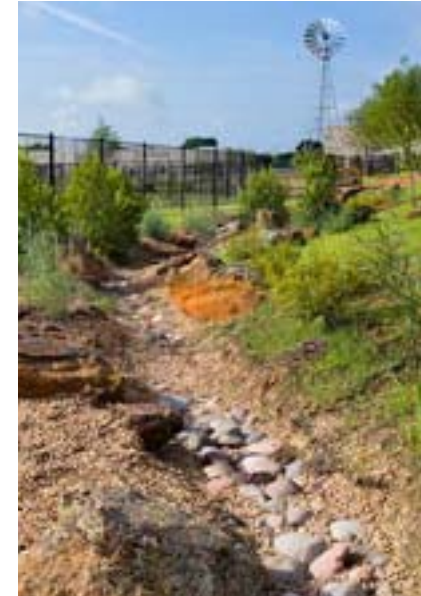
Fig 7-47 Parking area and bioswale system
