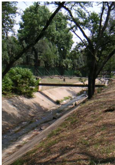
Fig 3-41 Occasional pedestrian bridge
