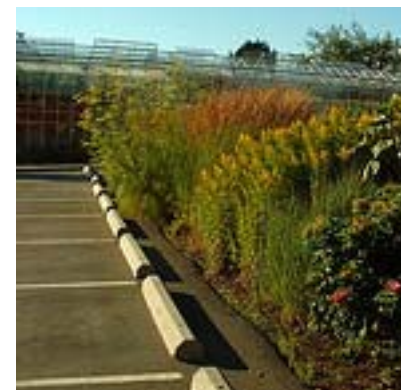
Fig 7-46 Parking area and bioswale system
