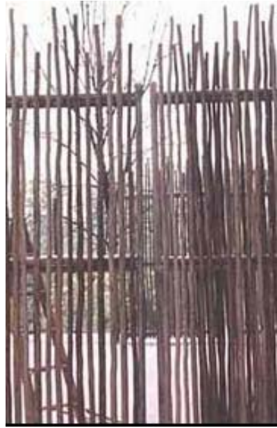
Fig 7-17 Wattle lathes screen
