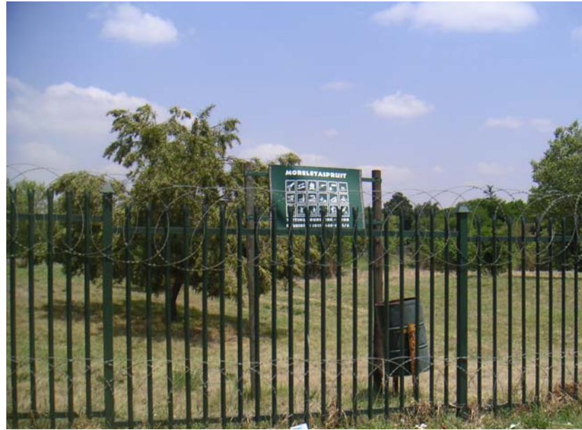
Fig 4-11 Palisade fencing and barbed wire.
