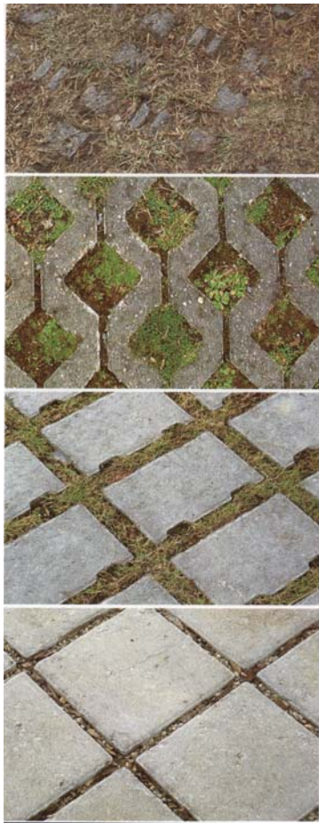
Fig 7-42 Permeable paving block
