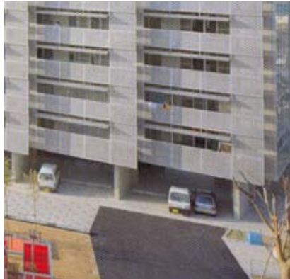
Fig 3-35 Slither housing - parking tucked underneath the building
