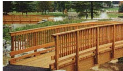
Fig 6-72 Timber foot bridge
