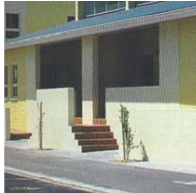
Fig 3-5 Royal Maitland covered entrances.
