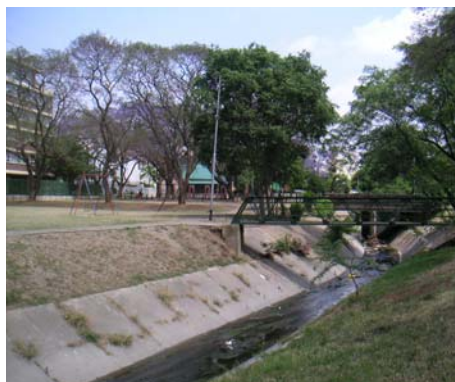
Fig 3-42 park space next to the spruit
