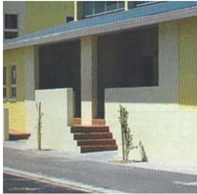
Fig 3-33 Royal Maitland covered entrances.
