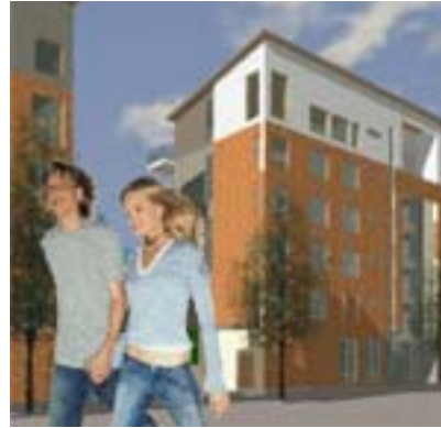
Fig 4-69 Plus home Project
