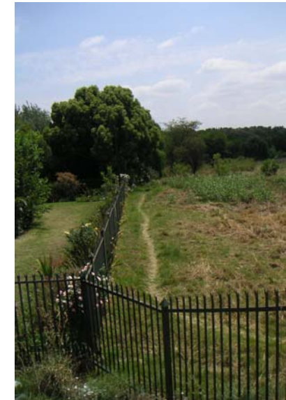
Fig 4-13 palisade fencing around the green strip.
