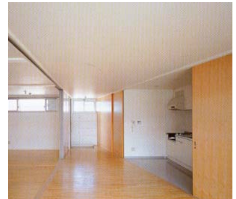
Fig 3-23 movable partitioning Slither Housing
