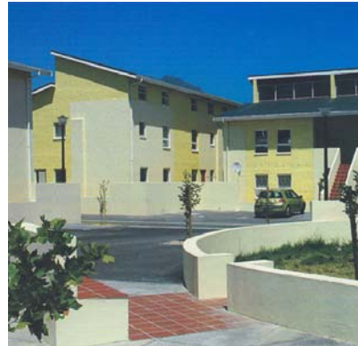
Fig 3-4 Royal Maitland playground square
