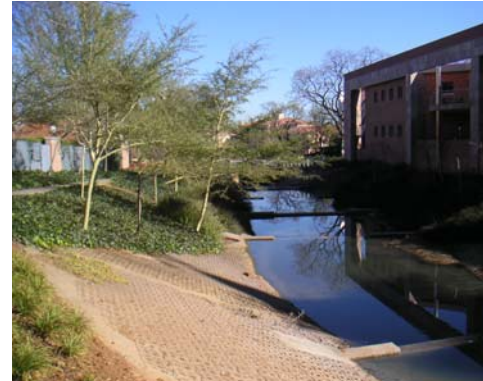
Fig 3-53 Concrete weir and rehabilitation of the river bank
