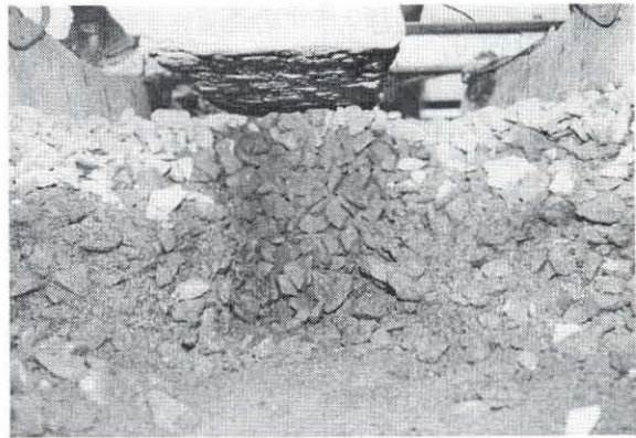
Clean ballast under sleeper
