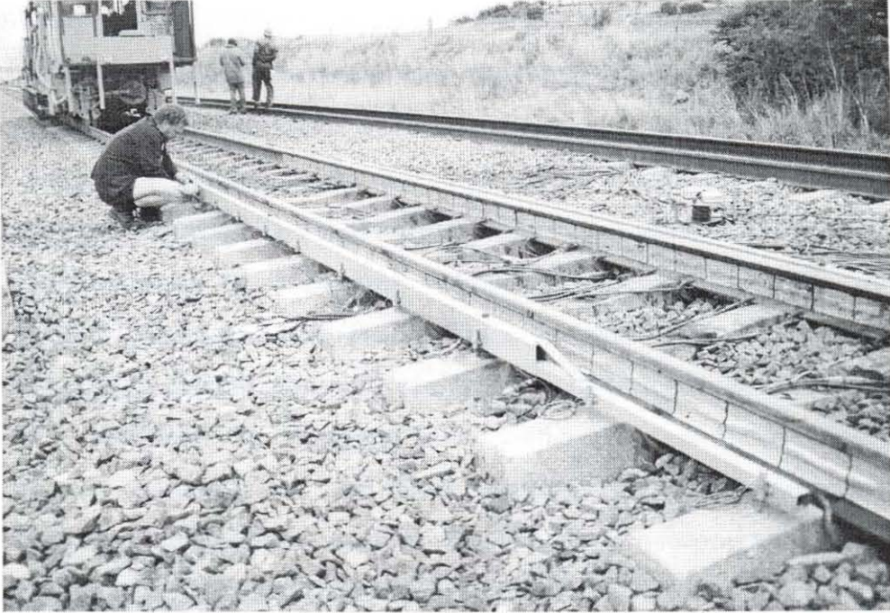
Figure 3.1: Instrumented test site.
