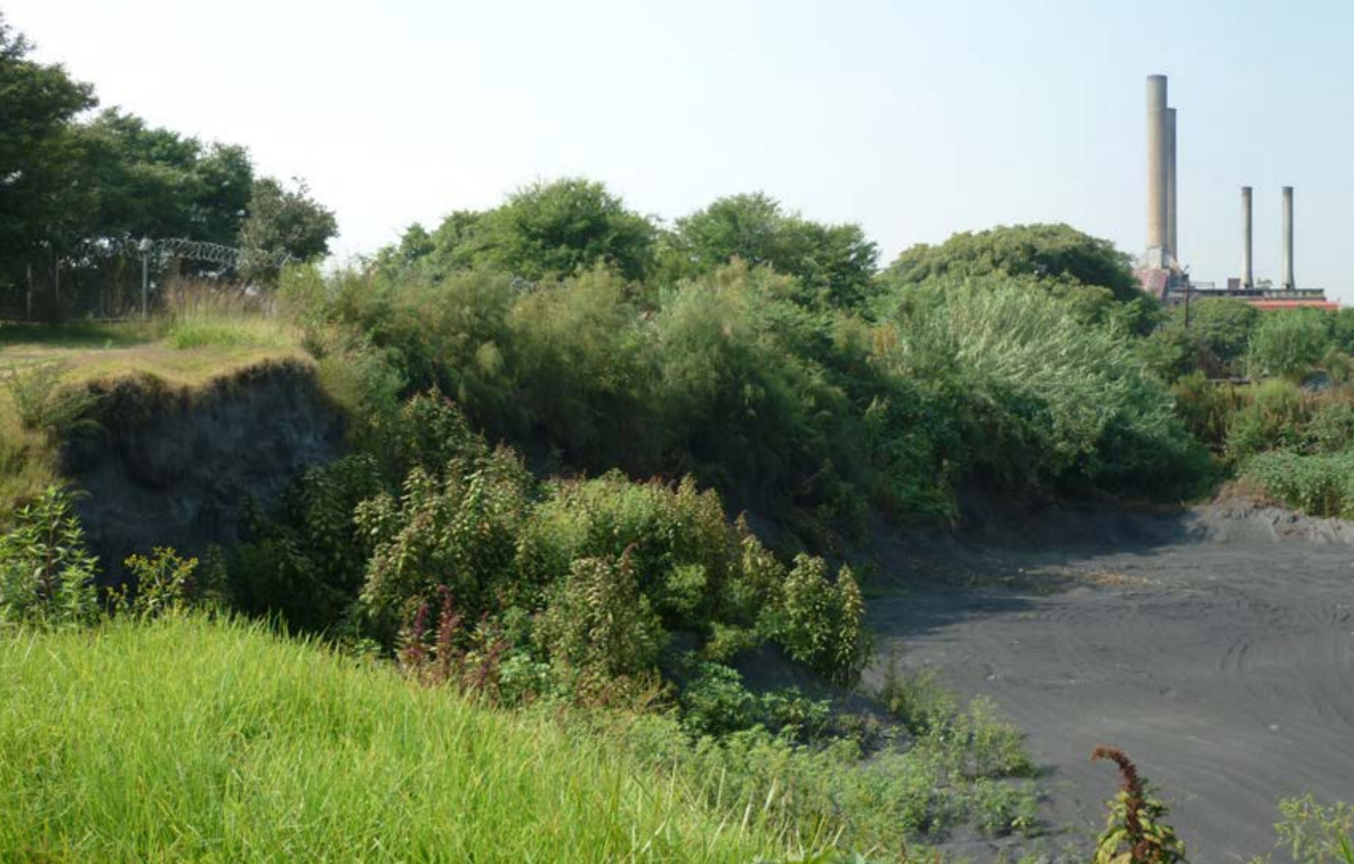
104 Fig:73. Panorama looking south at the eastern ash pond with the power plant in the background ( Author 2010)
