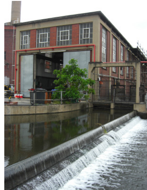
Fig:97. Pump house (Author 2010)
