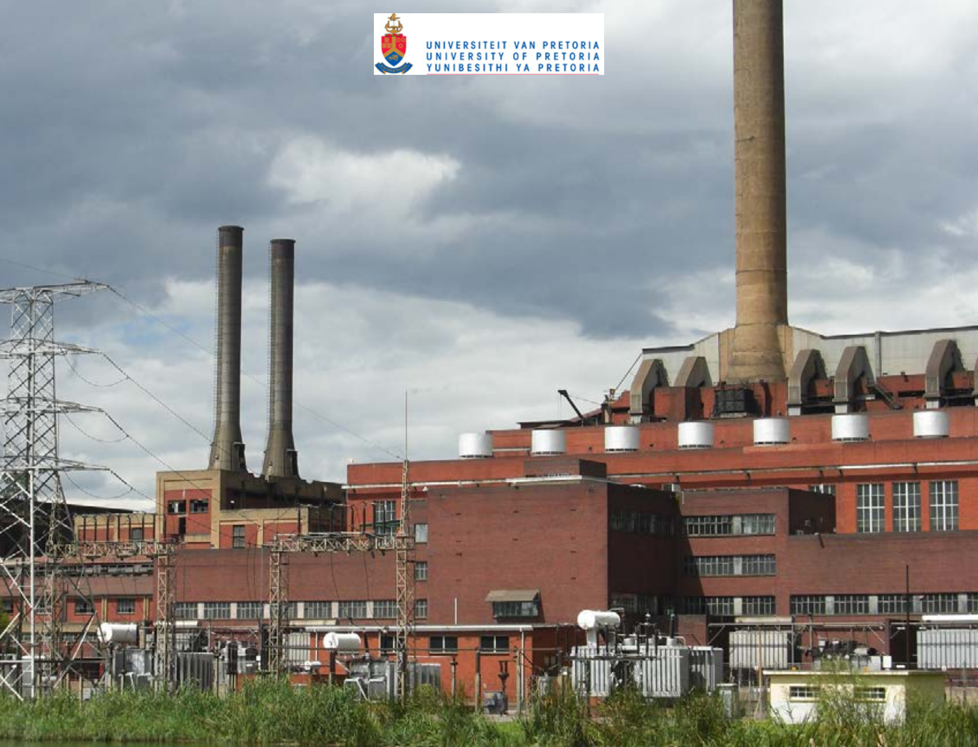
Fig:69. East ward view of power plant complex (Author 2010).
