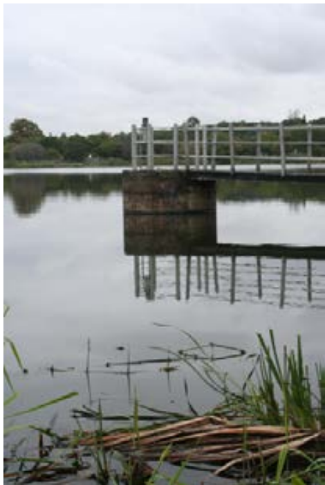
Fig:98. Water level meter (Author 2010)
