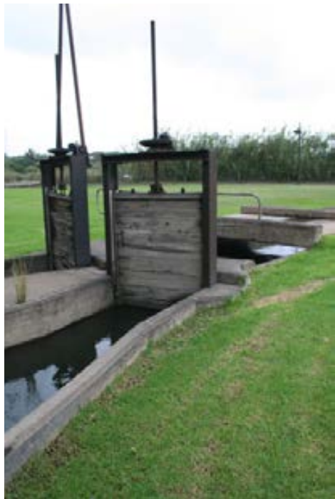
Fig:99. Canals and sluices (Author 2010)
