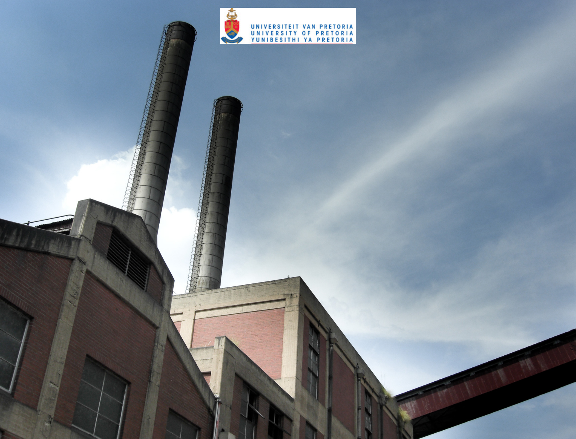
Fig:110. The old turbine hall 1938 (Author 2010)
