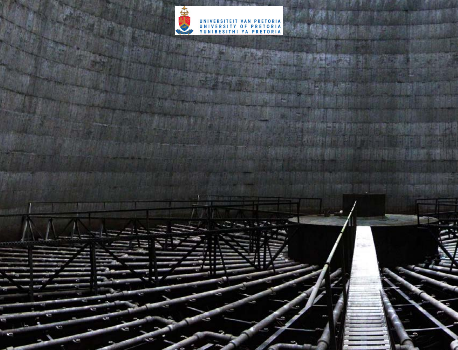
Fig:67. Inside one of the cooling towers (Author 2010).
