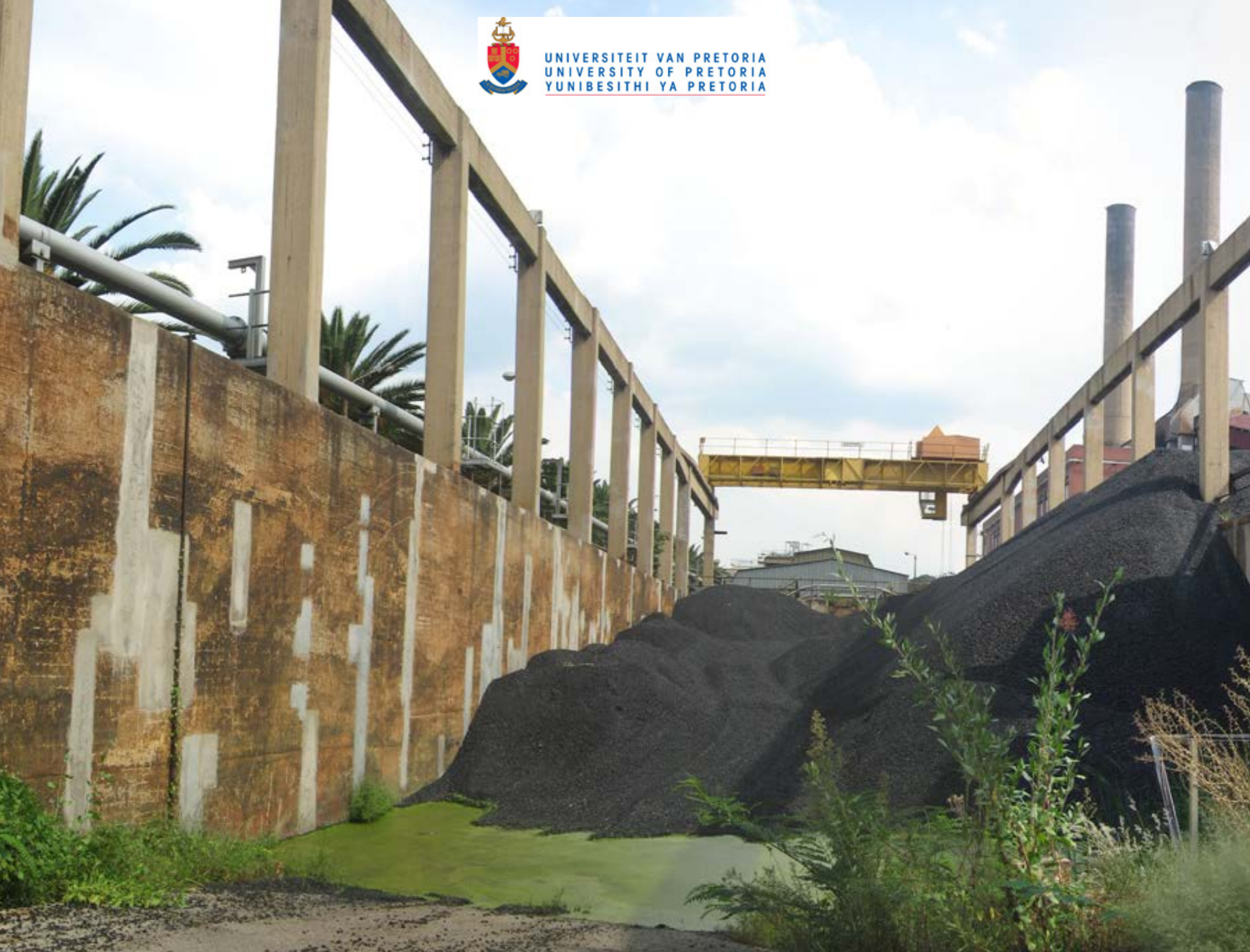
Fig:141. Inside bunker B (Author 2010)
