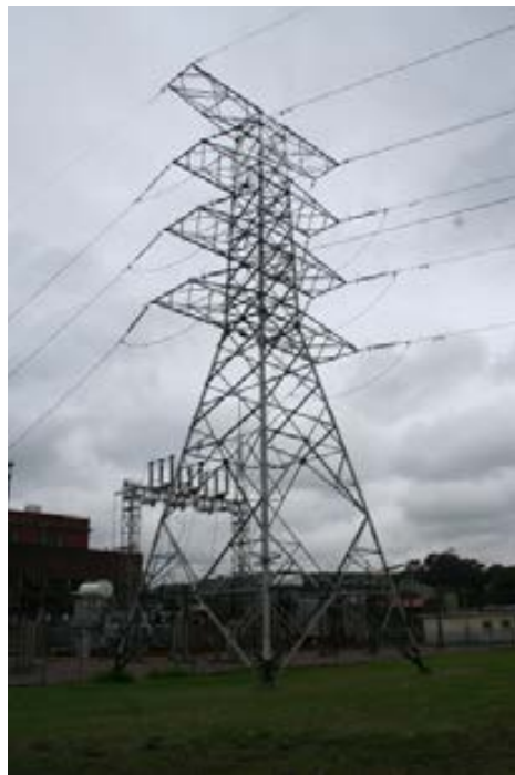
Fig:100. Electric pylons (Author 2010)
