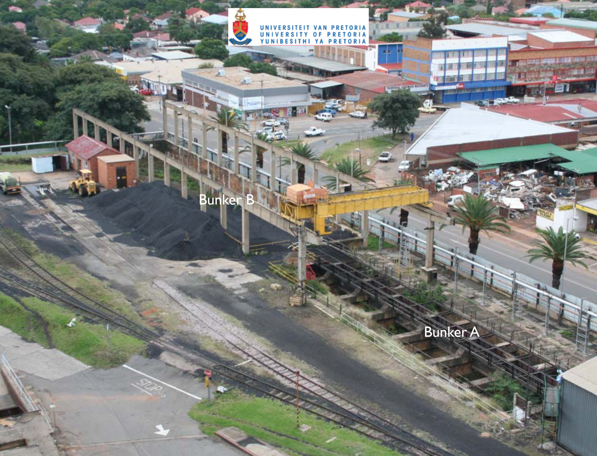
Fig:137. View of coal bunkers (Author 2010)
