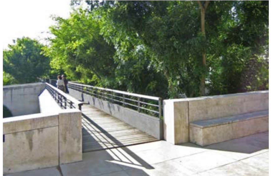
Fig:151. Raised walkways in Andre Citroen Park ( http://architypes.net/image/parc-andre-citroen-walkways-over-gardens )
