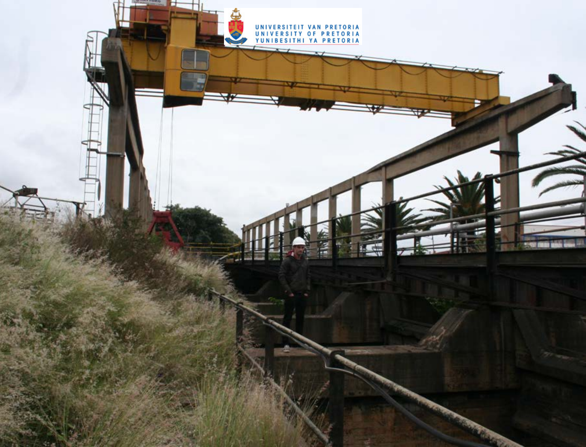
Fig:130. View of historic coal bunkers 1933 and 1945 (Author 2010)
