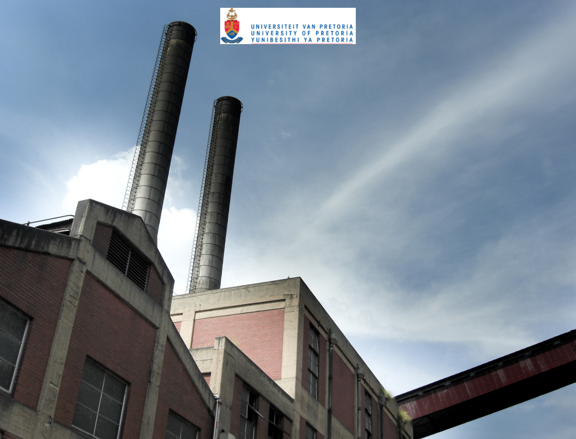
Fig:110. The old turbine hall 1938 (Author 2010)
