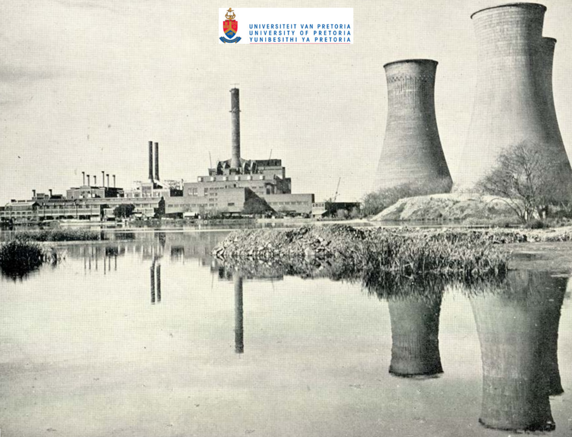
Fig:62. Historic photograph of power plant taken in 1952.
