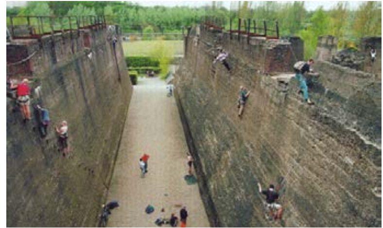
Fig:81. Ore bunker adapted for rock climbing (Reed 2006: 129)
