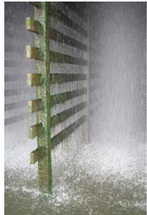
Fig:101. Under cooling tower (Author)
