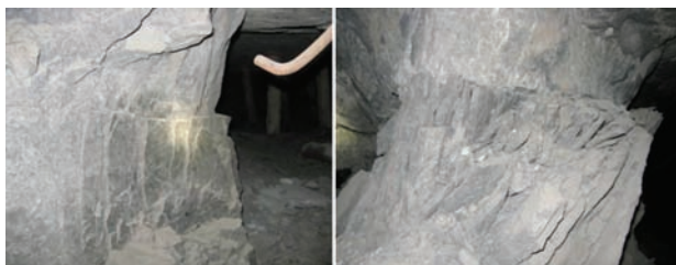
Figure 1—Example of a complex pillar failure mechanism. A weak horizontal calcitic joint is present in the UG2 pillar on the left, and this causes the pillar failure mechanism shown on the right
