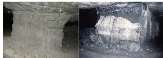
Figure 16—Examples of underground pillars with different pillar/host rock moduli. (a) Platinum mine pillar with modulus approximately similar to the host rock. (b) Coal mine pillar with modulus lower than the host rock (photograph courtesy of Prof. Nielen van der Merwe)
