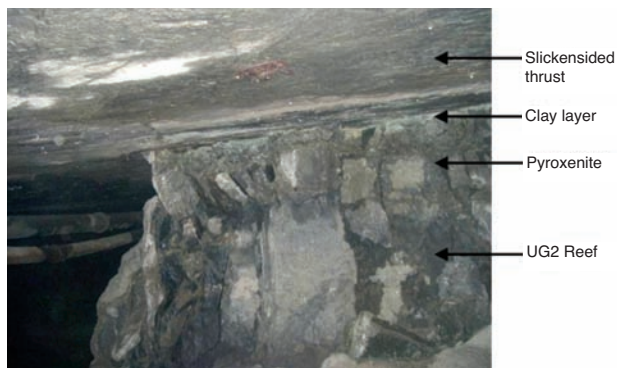
Figure 15—Typical pillar composition at Mine A (after Roberts and Clark-Mostert 37 )
