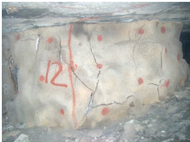
Figure 16—Pillar failure at Mine A after attempts to strengthen the pillars with shotcrete (photograph courtesy Dr Mike Roberts)
