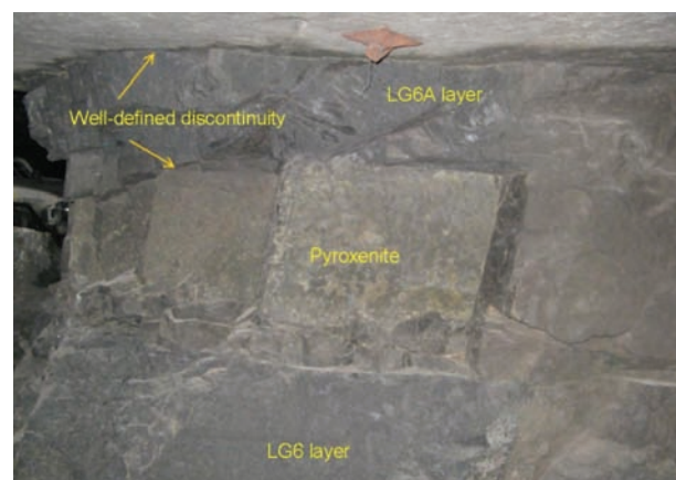
Figure 9—Typical multi-layer composition of pillars in the Bushveld Complex mines exploiting the LG6 and LG6A chromitite layers
