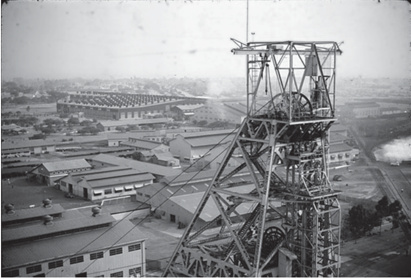
Mufulira Mine Selkirk Shaft head frame and hoist house, 1960. (From Northern Rhodesia Chamber of Mines Year Book, 1960 [Kitwe, 1961], facing p. 1.)
