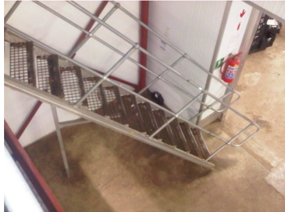
Figure 3: Top Photo of stairs leading to Print Room
