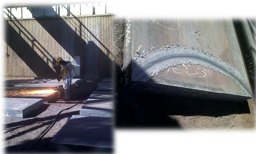
Figure 19: Inspection of slabs
