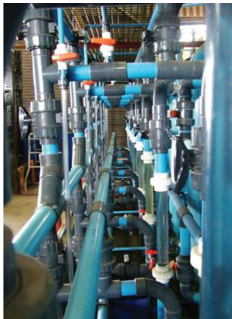
Figure 9: Ion Exchange columns (DOYLE, Dr Richard, 2009)
