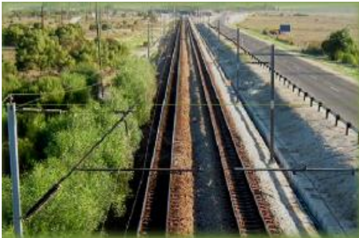
Figure 12: Coal export line Rail Track
