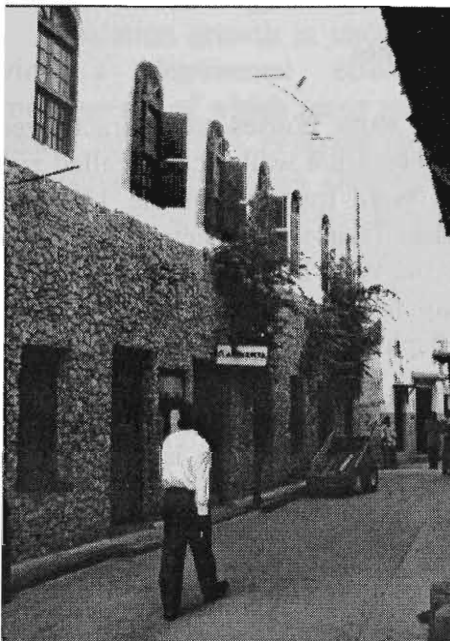
Figure 14. A rough finish with coral chips. character.
