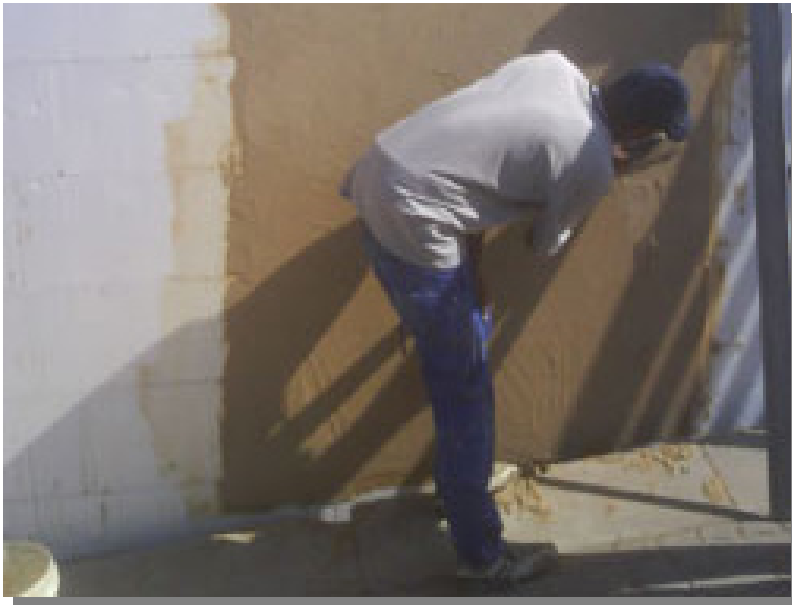
Figure 10 - Application of polyplast onto a wall. ( www.abpbuildingproducts.co.za )
