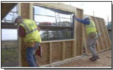
Figure 7 - OSB boards mounted against frame (osbguide2006:3)
