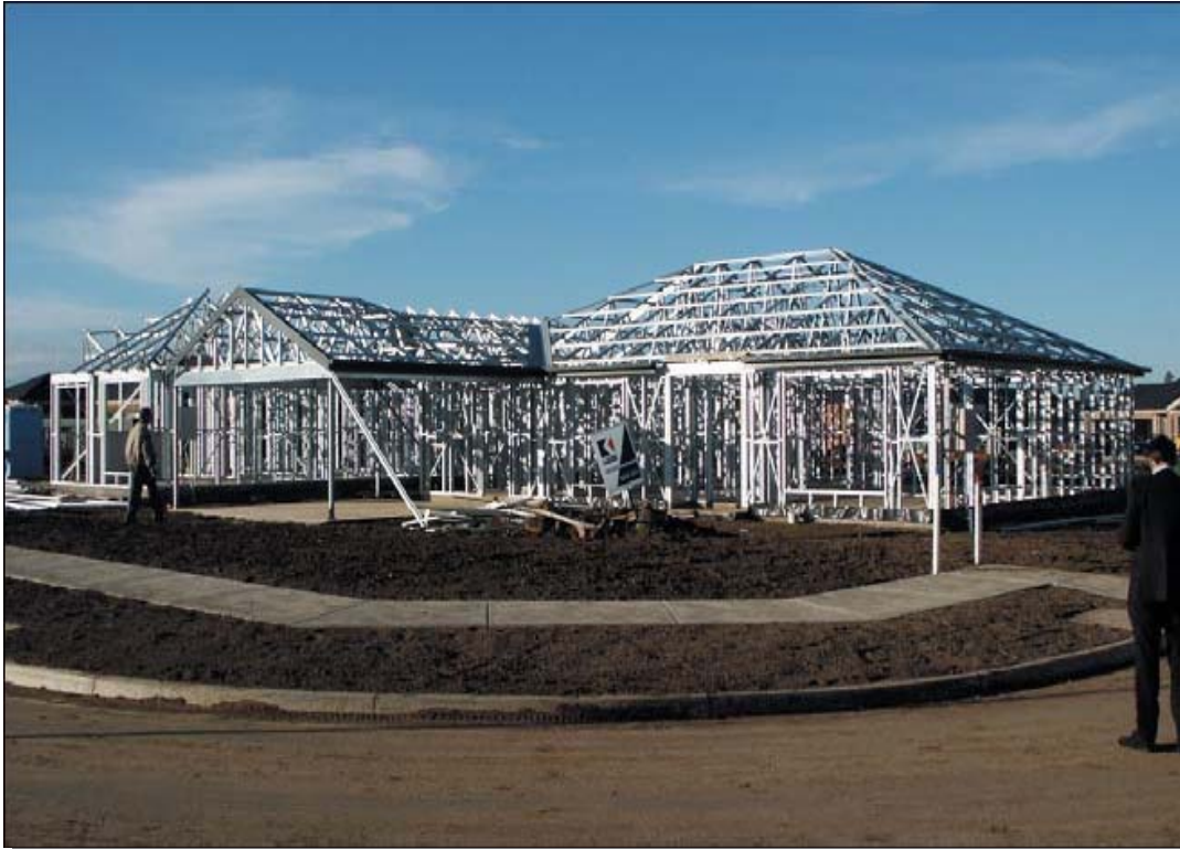
Figure 27- Framed wall house (www.steelhd.co.za)
