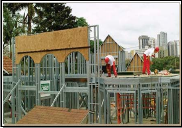
Figure 20 : Lightweight steel structure house being constructed (osbguide2006:5)
