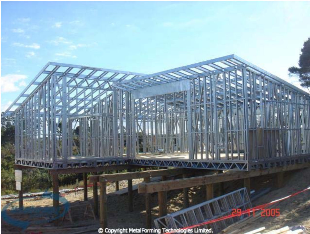
Figure 26- Framed wall System on site ( www.metalformingtechnologies.com )
