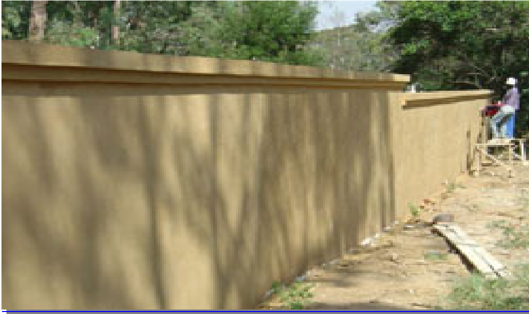
Figure 11 - Finishing of Polyplastered wall ( www.abpbindingproducts.co.za )
