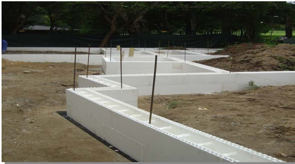
Figure 9- Polyblocks on site (Polyblock leaflet: 3)
