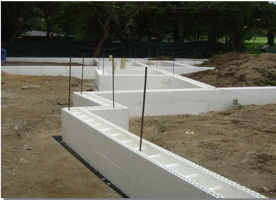
Figure 19 – Polyblocks on site (Polyblock leaflet: 3)
