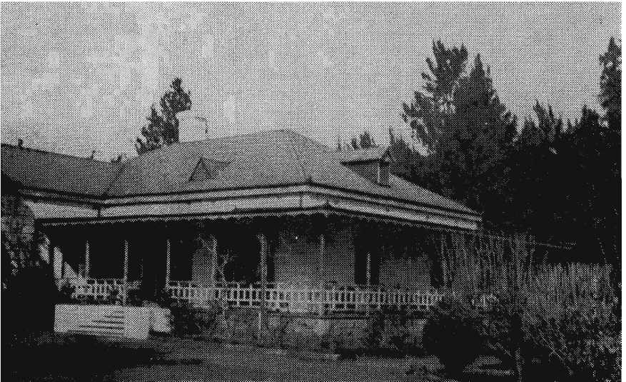
Farm House. View from the North.
