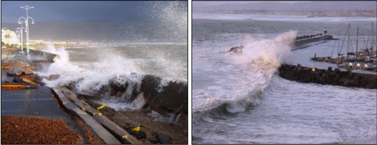
Figure 5: Storm breaching a seawall and overtopping (Cape storm: Sept'08) - examples of existing problems likely to worsen due to climate change (Photos: A Theron)
