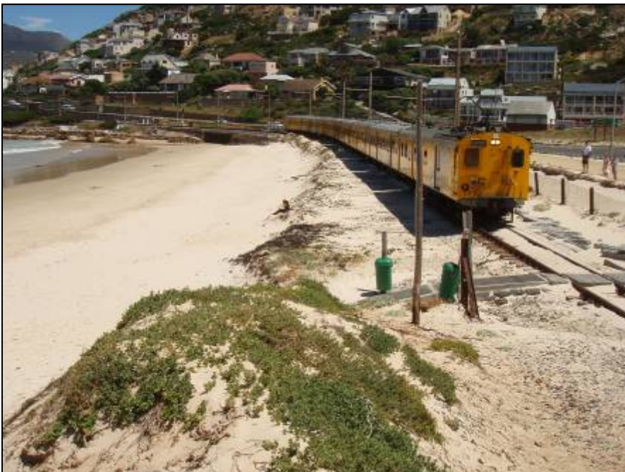
Figure 6: Present SA example of railway line located too close to sea (Photo: A Theron)
