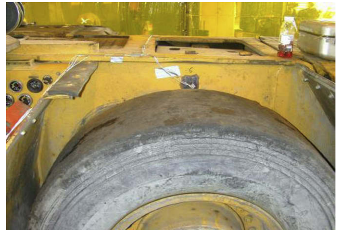
Fig. 8. Strain gauges above wheel-arch (channel 4).
