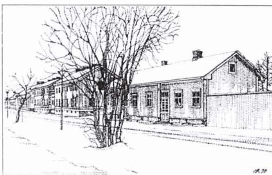
Figure 1: Log houses of wooden towns are one- or two-storey. Their roofs are steep and they have a high base.
