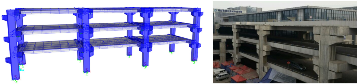
Figure 3: Prototype and finite element model of the framed 3-layer overpass bridge
