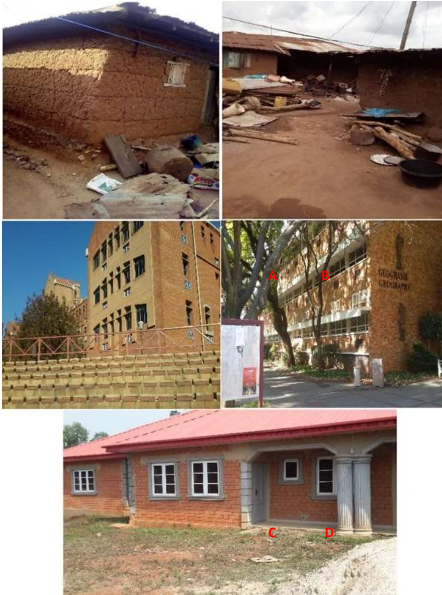
Figure 1: Different faces of earth bricks in building construction. (A&B) Ebira Farm Settlement in Nigeria, (C&D) Departments of Economics and Geography (fired bricks), University of Pretoria, (E) Catholic Mission House in Nigeria (CEB).
