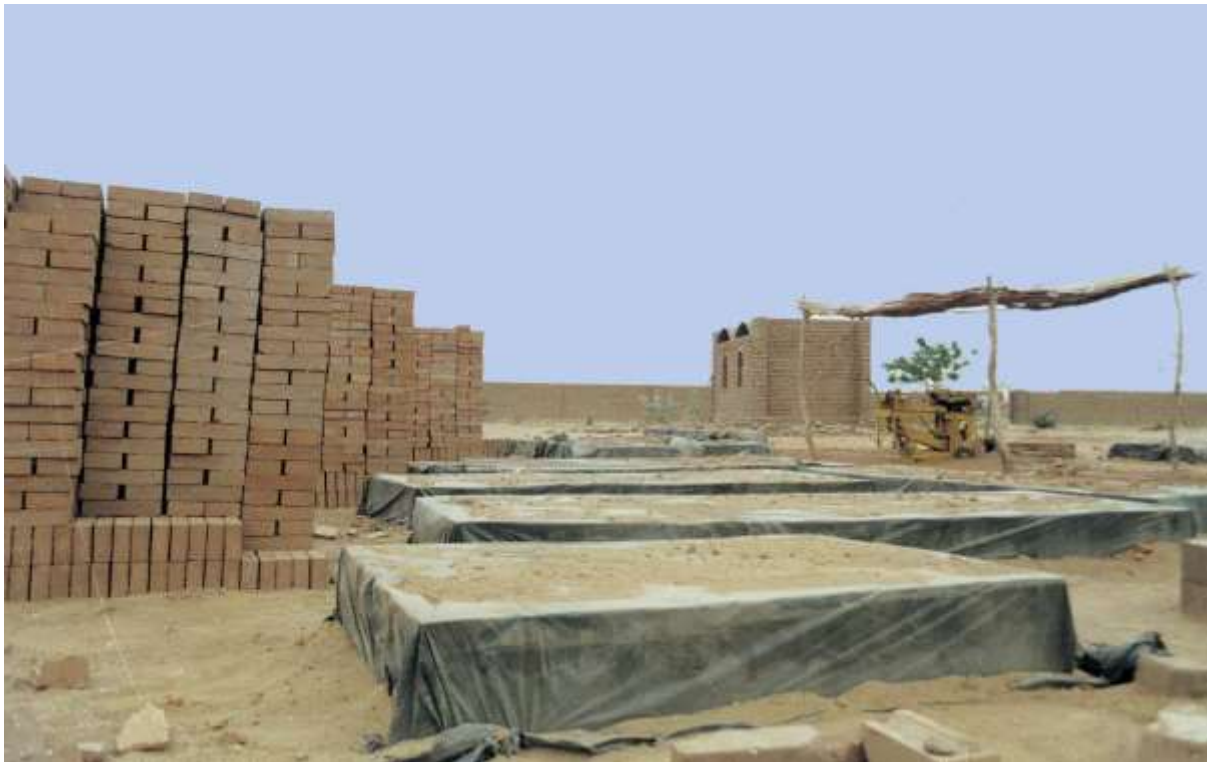
Figure 6: A Curing Process of CEB. (After, Adam and Agib, 2011)
