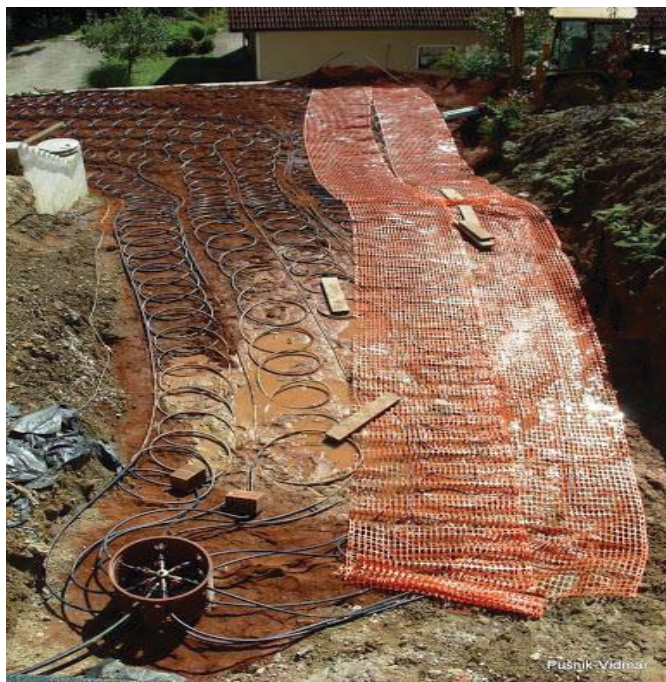
Figure 2 Ground source heat collector
