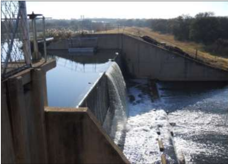
Figure 29: Zeekoegat WWTW outlet structure
