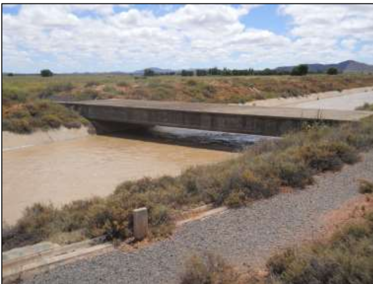
Figure 19: Pedestrian bridge across the Teebus canal, SA
