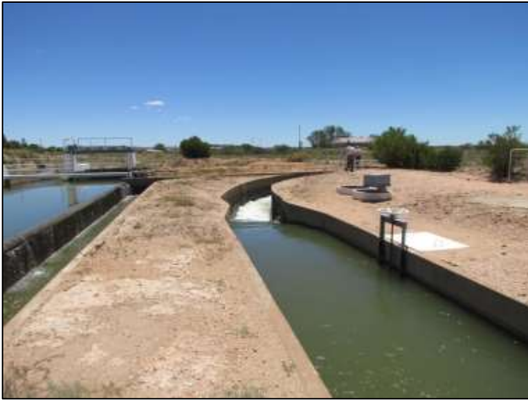
Figure 17: Example of a diversion structure in the Boegoeberg Irrigation Scheme, SA [29]
