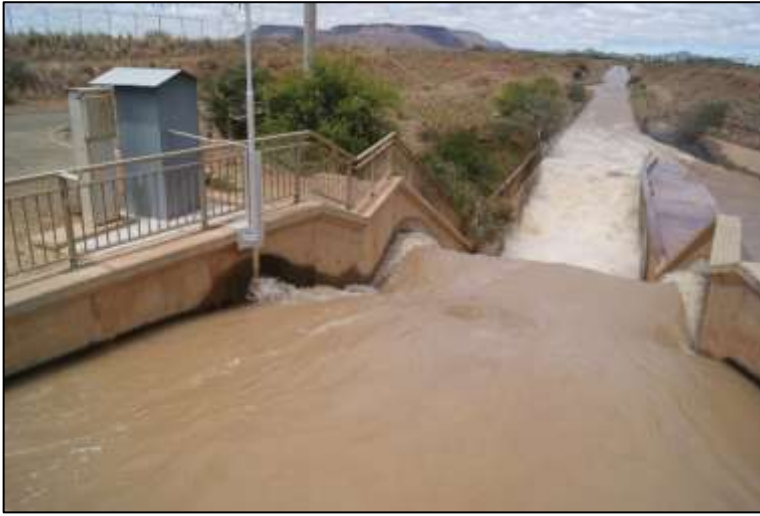
Figure 20: Flow gauging telemetry system at the Teebus canal, SA
