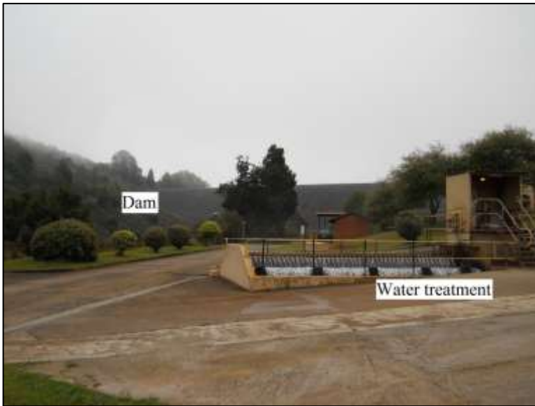
Figure 26: Ebenezer Dam and water treatment works
