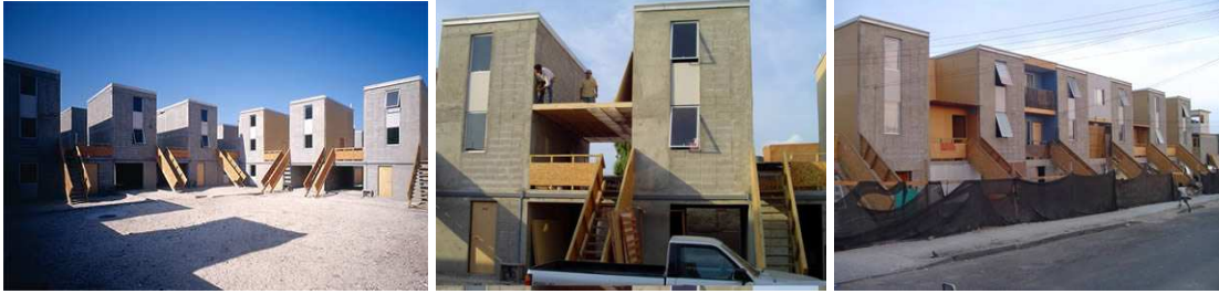
Figure ? Quinta Monroy just after completion Figure ? Occupant additions beginning Figure ? Some additions completed
