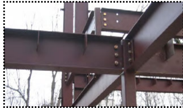
Figure 07 | 3. steel beams on site
