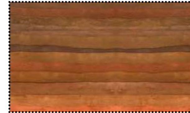
Figure 07 | 7. sirenwall rammed earth
