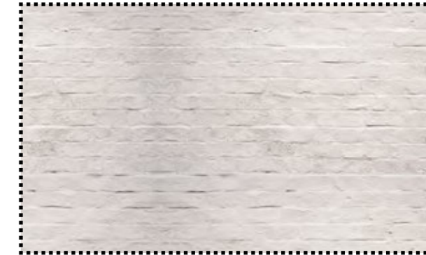
Figure 07 | 8. plastered adobe bricks
