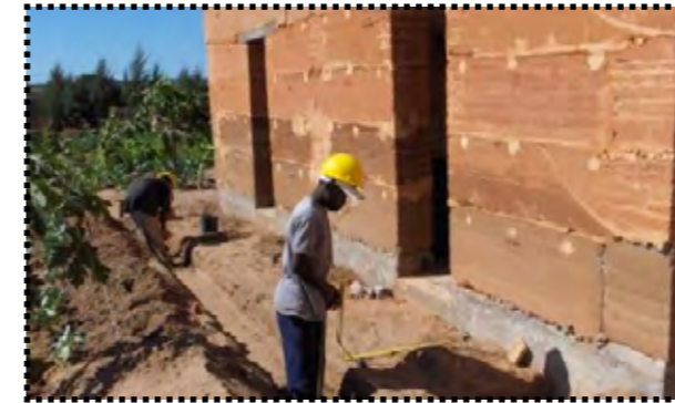
Figure 07 | 6. earth construction underway
