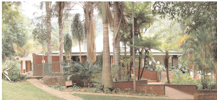
Fig. 2.4.6.1.1.1 Existing farmhouse, southeast elevation
