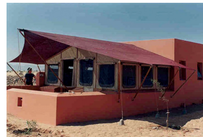
Fig. 5.4.5 North-western view with higher eastern wall
