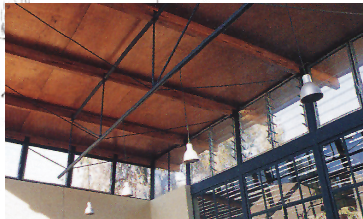
Fig. 5.3.3 Glass wall and clear-storey windows
