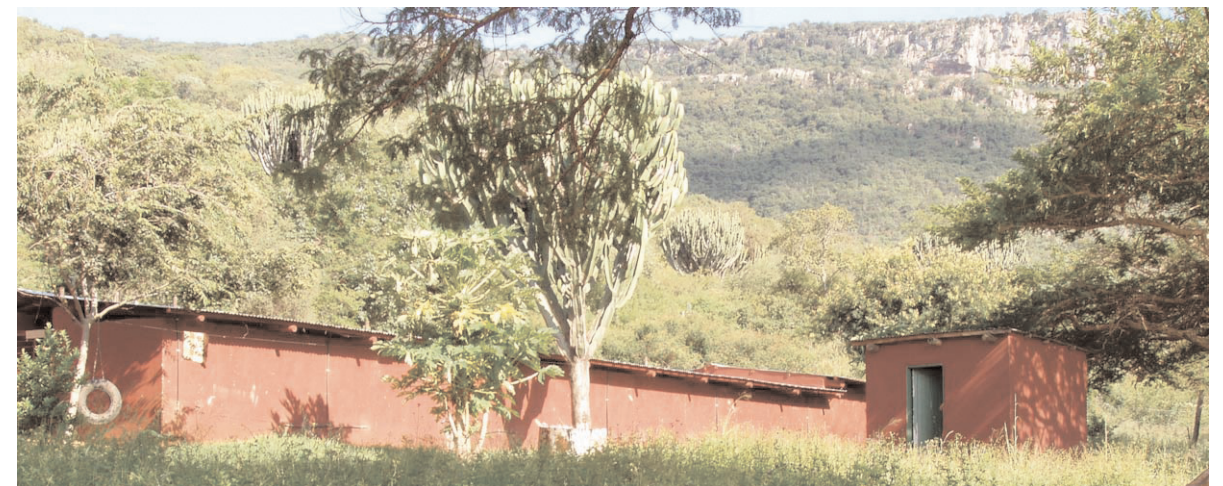
Fig. 2.4.6.1.1.6 North eastern view of existing swinery and storeroom
