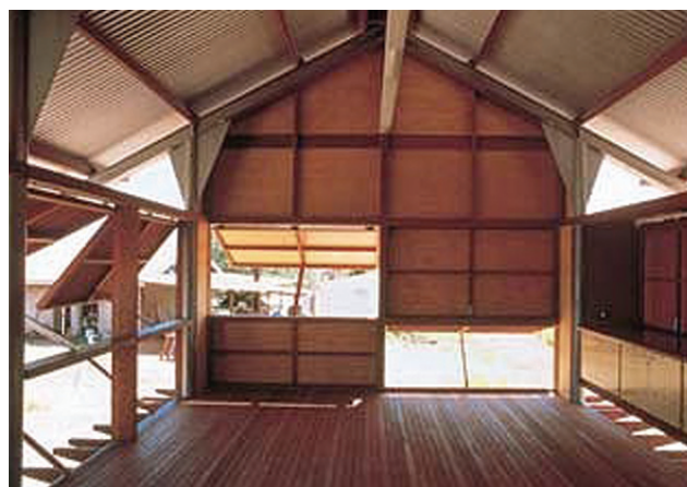
Fig. 5.2.4 Movable cladding panels
