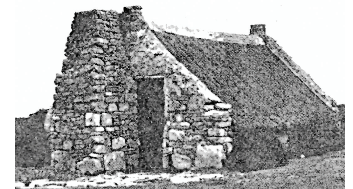
Fig. 2.4.6.1.2.6 'Kapsteilhuis' lifted onto low walls
