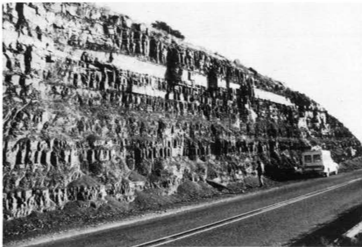
Plate 3: Variety of rock types and qualities in road cutting at Nelspoort near Beaufort West
