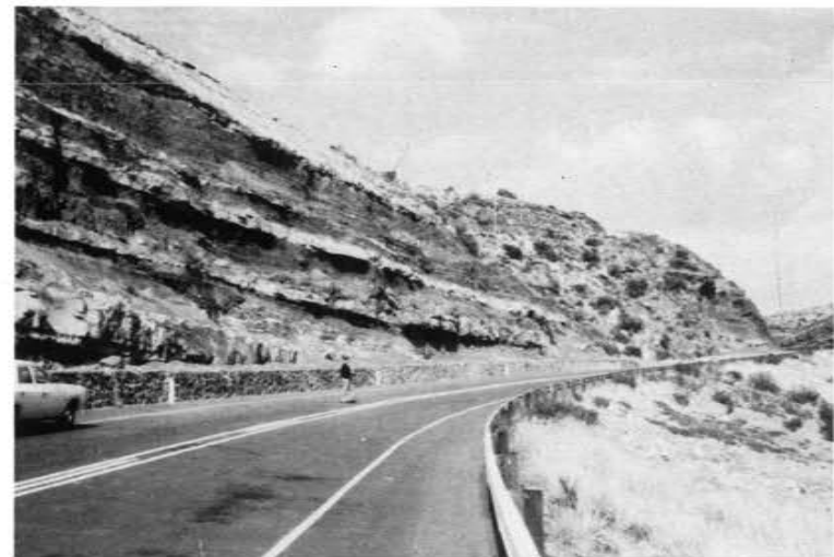
Plate 4: Erosion of mudstone of the Elliot Formation between resistant sandstone layers on the road between Lady Grey and Barkly East
