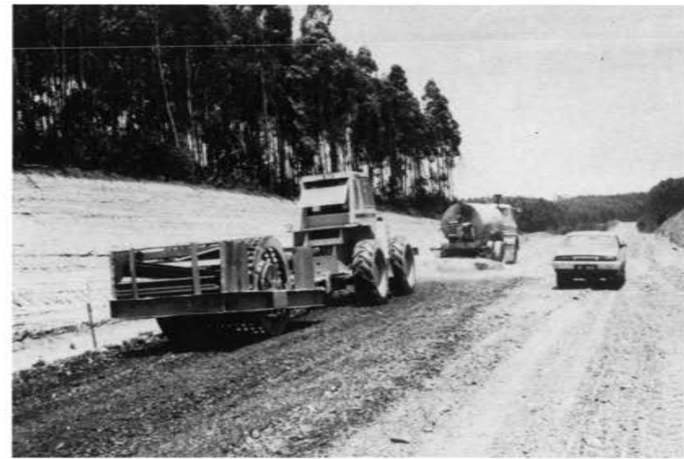
Plate 8: Grid roller being used for construction with mudrock on road between Mooi River and Greytown
