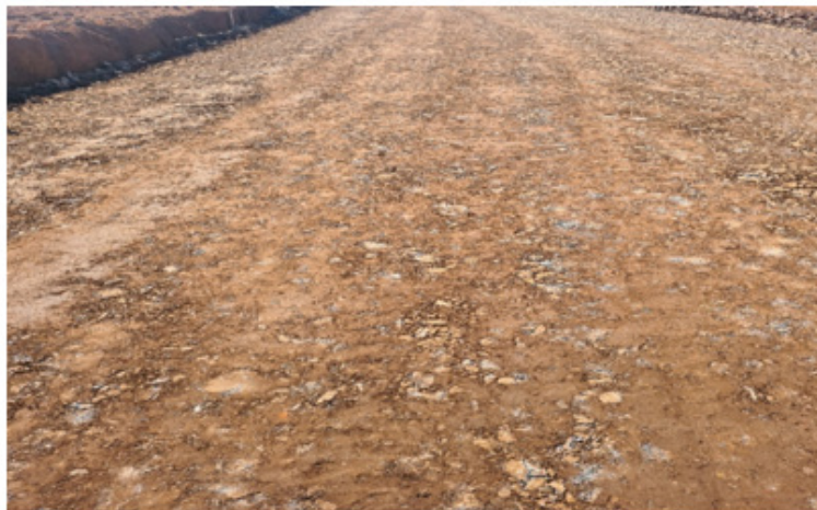
Figure 3: Layer completed after compaction
