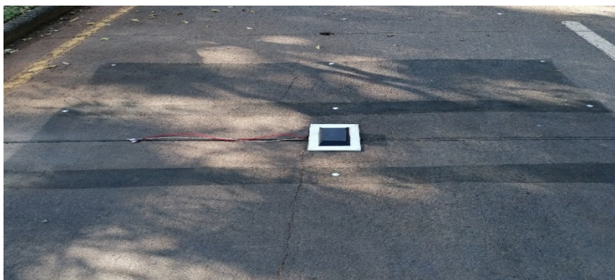
Figure 5: RFID reader in-road setup. Source: Author
